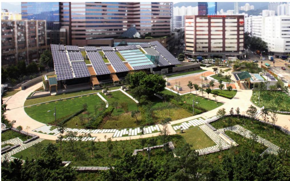
Fig. 4.2.9. CIC Zero Carbon Building (Ronald Lu and Partners)
