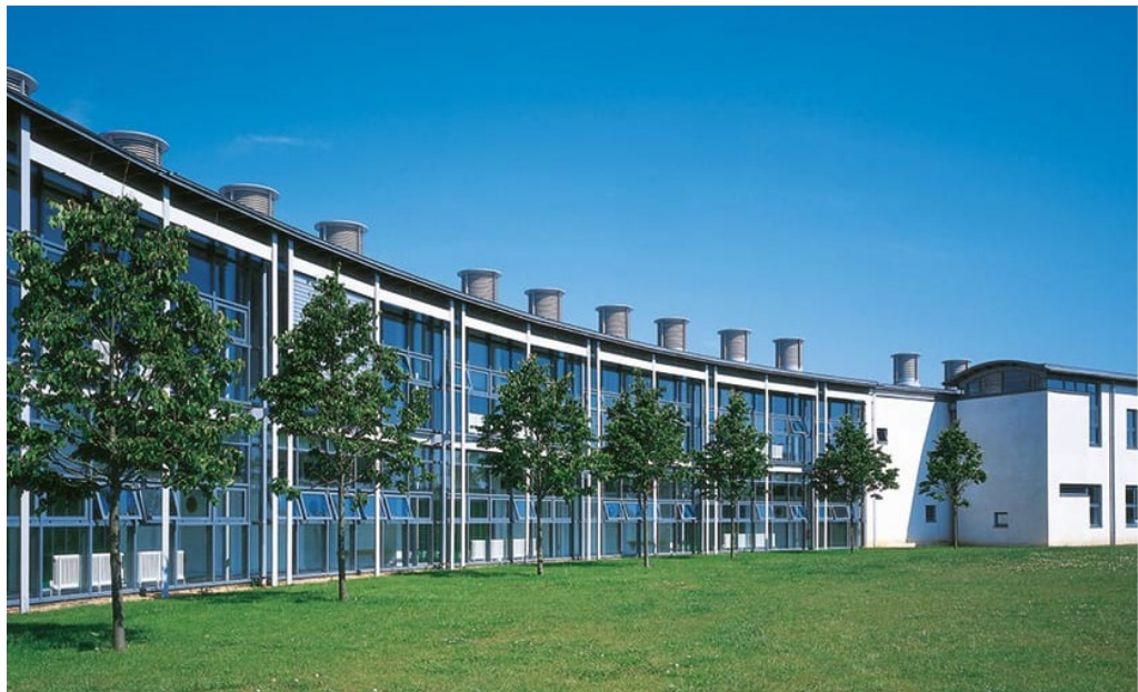
Fig 4.2.7. Haute Vallee School (PBL Architects)
